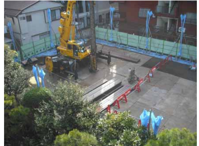
Situation of the construction site
