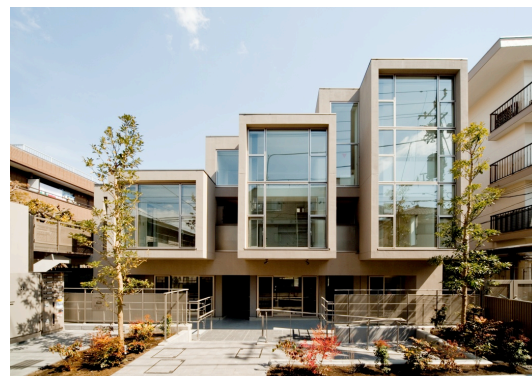
CHISUIKAN, the world's first building installed with 3-D isolators
